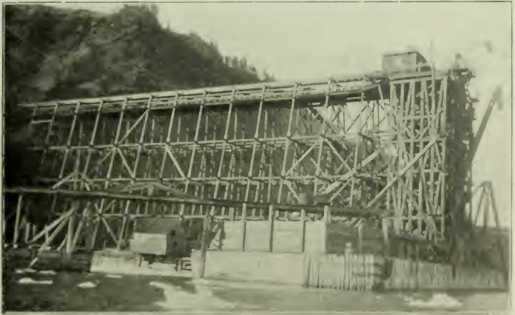
Side View of Shipping Pier, at Wabana Iron Mines.
